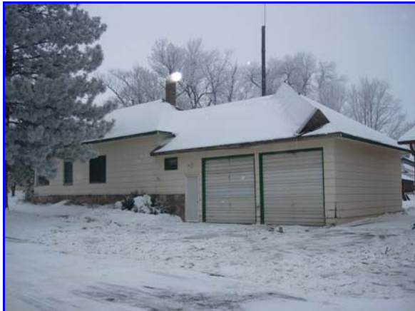
2-Car Attached Garage
